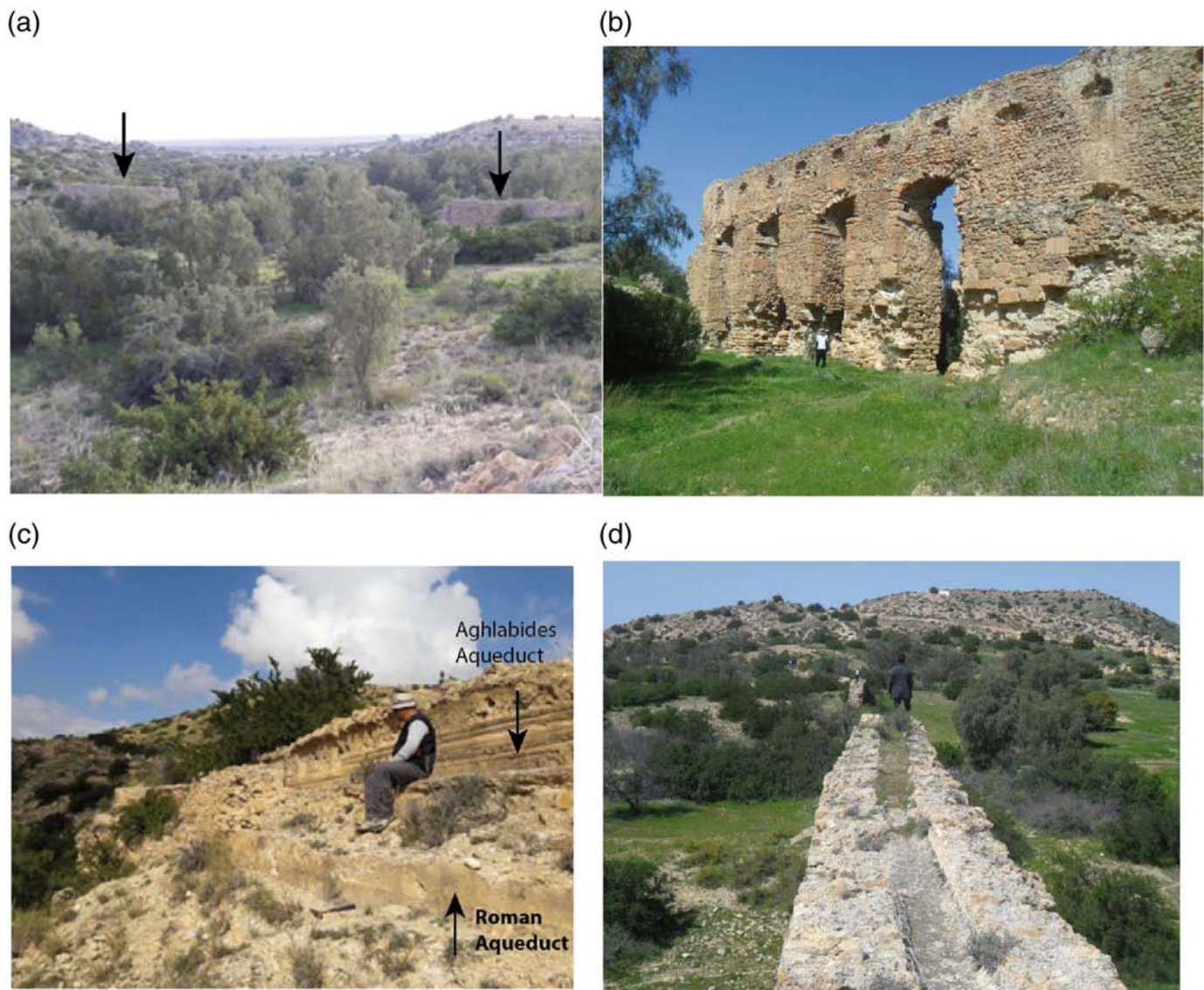
Figure 8. (a) The aqueduct bridge with its edges (arrows) crossing the Cherichira River; (b) ~25-meter-high aqueduct bridge with 2.9 × 2.9 m pillars built during the Roman time in Tunisia (146 B.C.–A.D. 423) and the Aghlabides period (A.D. 800–909); (c) the Roman and Aghlabides Aqueduct exposures; and (d) top of the aqueduct with a canal on the bridge. The color version of this figure is available only in the electronic edition.
