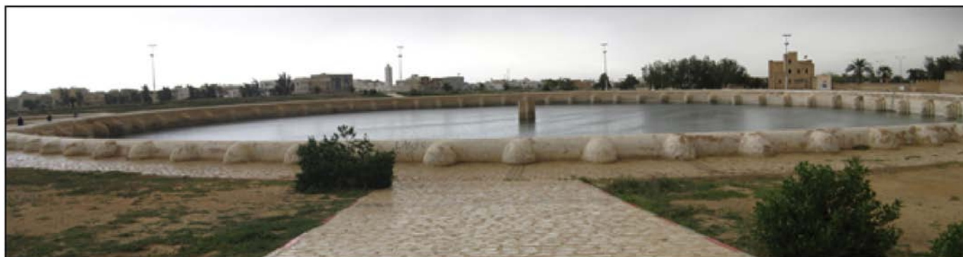
Figure 3. Open air cistern also called Feskiya of Bab Tunis in Kairouan. Water reservoirs like this were built in early A.D. 860 due to a water shortage. The diameter is almost 130 m, and it is about 5 m deep. The color version of this figure is available only in the electronic edition.
