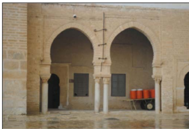
Figure 4. Two retrofitted arches in the Kairouan Great Mosque. The two retrofitted arches show different structures with the lower left structure and distorted right arch. Pillar tops are not at the same level, and the two structures are clamped with three iron hooks. The color version of this figure is available only in the electronic edition.
