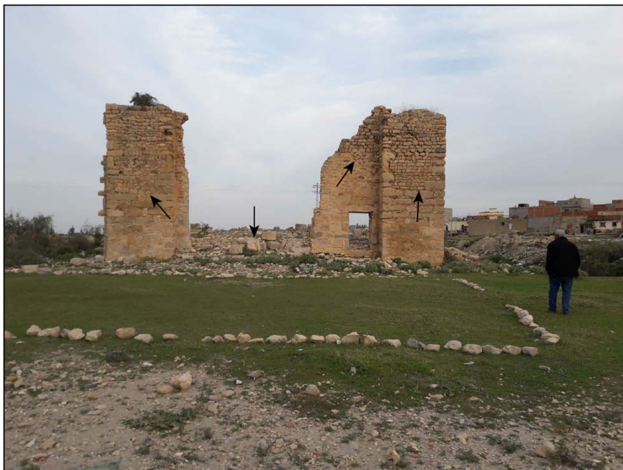
Figure 6. Damaged Roman city of Cululus (now Ain JIoula, see location in Figs. 1 and 2a,b). Arrows on frontal wall show the different building stones with evidence of reconstructions and
